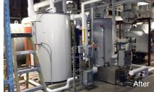
"Since the heat exchangers and storage tanks could be separated, PVI's Cobrex units could easily be put in to the existing space. Although access to the space in the mechanical room was difficult, no doors, existing equipment, or ductwork had to be moved to get the new units into place." Mark Reinhardt, Specified Design Consultants.
